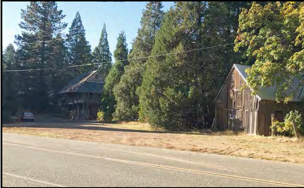
Photo 1. Exterior view, Mountain House Historic District, Overview, looking southwest (Photo by Corri Jimenez).
