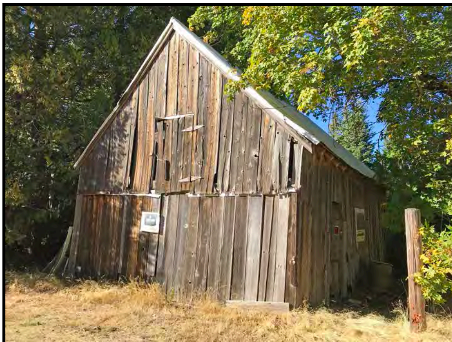
Photo 8. Exterior view, Mountain House Historic District, Barn, looking northeast (Photo by Corri Jimenez).
